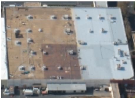
**SOLUTION:** Spray Polyurethane Foam Roof System. The removal of the existing 60,000 sq ft BUR roof and application of the SPF roof with base coat was completed in just 7 days - making the building water tight with increased energy efficiency.
