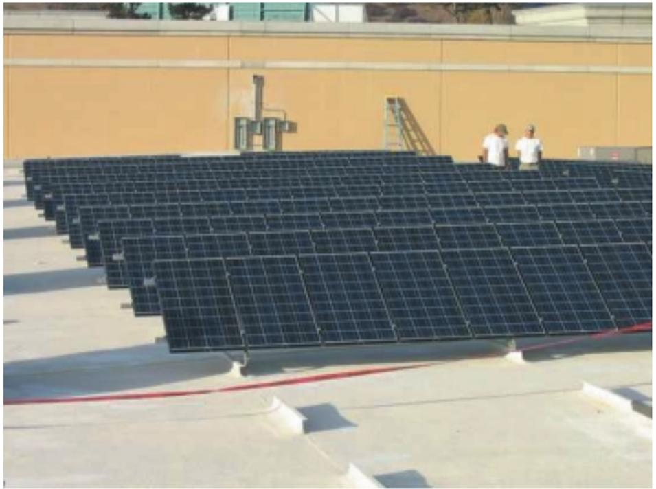
***Replacing heavy, inefficient BUR with lightweight, watertight SPF made it possible to install a Photovoltaic solar system without requiring costly structural upgrade.***
